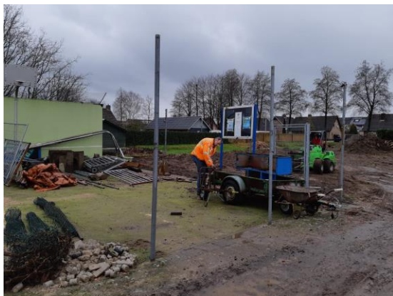
Start montage boarding: 104 gaten boren in asfalt en klinkers.
